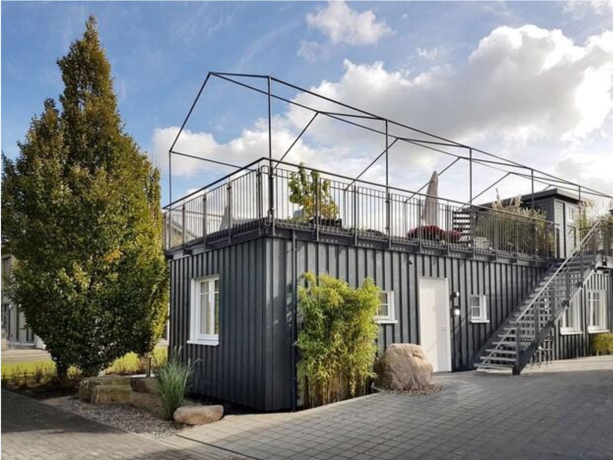
Fig.: Green Living Space a cooperation project of the project partners SchwörerHaus, IKEA Germany
